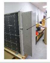
**NOTE:** Wind Blockers are used to prevent direct wind exposure to the heat exchanger. Windscreens are needed for the operation where the ambient temperature falls below -5° Celsius.
