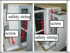
4. Secure lower safety string to lower left side of cabinet with existing cabinet screw. Secure upper safety string to top panel with existing cabinet screw.
