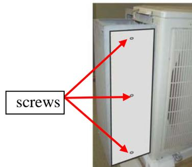
Note: Windscreens are needed for operation where the ambient temperatures fall below -5°C.
