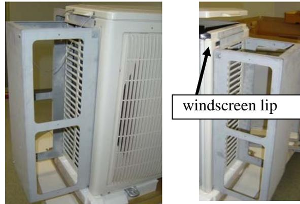
3. Align wind blocker to pre-drilled holes on the side windscreen. Attach wind blocker to the side of windscreen where there is direct wind exposure. Use screws provided.
