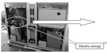
3. Remove the wires that are secured to the frames,
