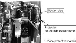
6. Place protective materials on the insulation lining compressor cover and on the compressor suction pipe to protect them from the torch flame, debraze the pipe, and replace the compressor.
