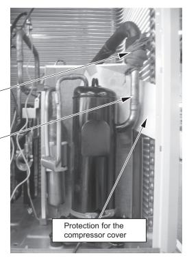
Place protective materials on the insulation lining of the compressor cover and on the sealing material on the compressor suction pipe to protect them from the torch flame, debraze the pipe, and replace the compressor.
