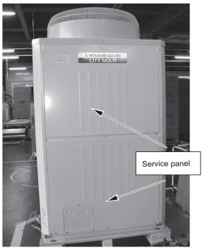
1. Remove both the top and bottom service panels (front panels).
