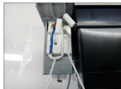
Thermal fuse Terminal plate
