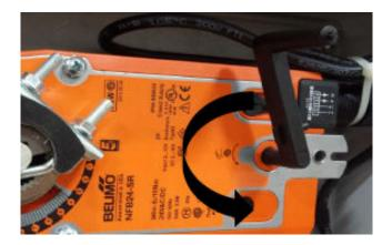
Step 5. Lock the motor in the 85 degree position.
