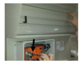
Step 8. Ensure that the end of the shaft is flush to the edge of the clamp black surface as shown.
