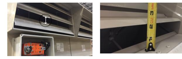
Step 5. Once the louver spacing is adjusted properly, release the locking mechanism on the actuator. The louvers should return to their default open position.
