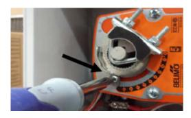
Step 2. Slide the mechanical stop to approximately 65 degrees (between the "6" and "7" marks) and tighten the screw, making sure the locating teeth on the stop are engaged into the actuator motor teeth.
