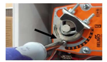
Step 1. Loosen the Philips head screw for the mechanical stop.
