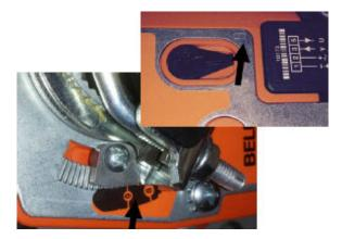
Step 6. Close the blades by hand and insert the crank handle under the damper blade near the screws as shown to ensure it is open approximately 1/4 inch at 85 degrees.
