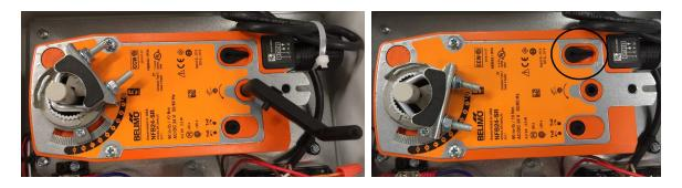
Step 4. Check the louver angle alignment in this position using a tape measure or other device. The gap between louvers should be 2.0". If the gap between louvers differs by more than 1/8", repeat steps 2 and 3 using a differing mechanical stop angle until acceptable louver spacing is achieved. See image below for measurement example.
