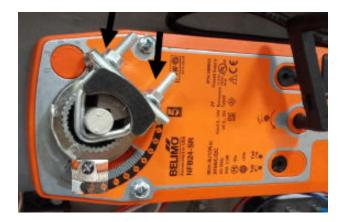
Step 4. Using the crank handle turn the motor counterclockwise until the indicator snugs against the stop at 85 degrees.
