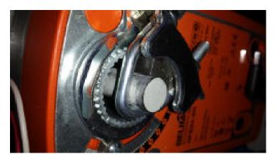
Step 9. Slightly crank the handle to release the motor. The damper will return to the open position.
