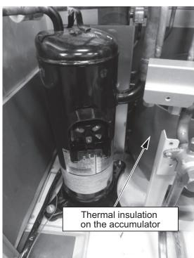
Remove or protect the wiring around the compressor and the thermal insulation on the accumulator, unbraze the pipe from the compressor, and replace the compressor. Follow the procedures below to remove the compressor components and replace the compressor. Reassemble them in the reverse order after replacing the compressor.
