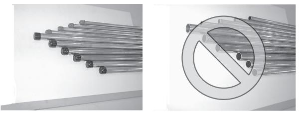
Both ends of the pipes should be sealed until just before brazing. Keep elbow pipes and T-joints in plastic bags.
