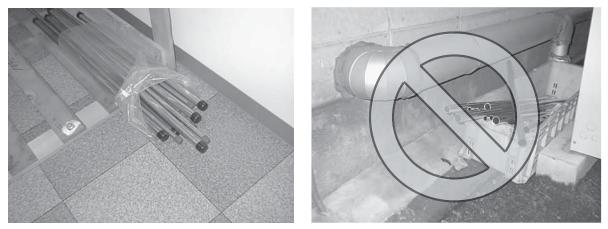
Store the pipes to be used indoors. (Warehouse at site or owner's warehouse) If they are left outdoors, dust, dirt, or moisture may infiltrate and contaminate the pipe.
