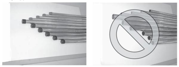
Both ends of the pipes should be sealed until just before brazing. Keep elbow pipes and T-joints in plastic bags.
