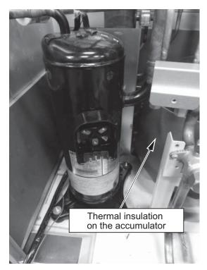
5. Remove or protect the wiring around the compressor and the thermal insulation on the accumulator, unbraze the pipe from the compressor, and replace the compressor. Follow the procedures below (Steps 1 through 4) to remove the compressor components and replace the compressor. Reassemble them in the reverse order after replacing the compressor.
