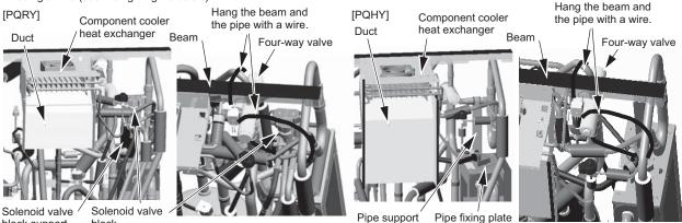
Solenoid valve block support block
