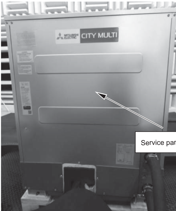
1. Remove the service panel (front panels).
