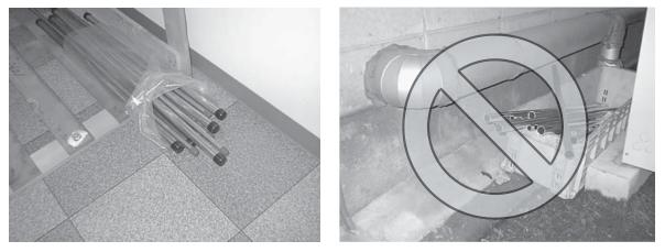
Store the pipes to be used indoors. (Warehouse at site or owner's warehouse) If they are left outdoors, dust, dirt, or moisture may infiltrate and contaminate the pipe.
