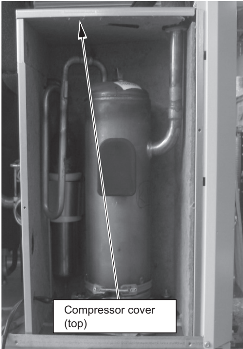
4. Remove the compressor cover (top).
