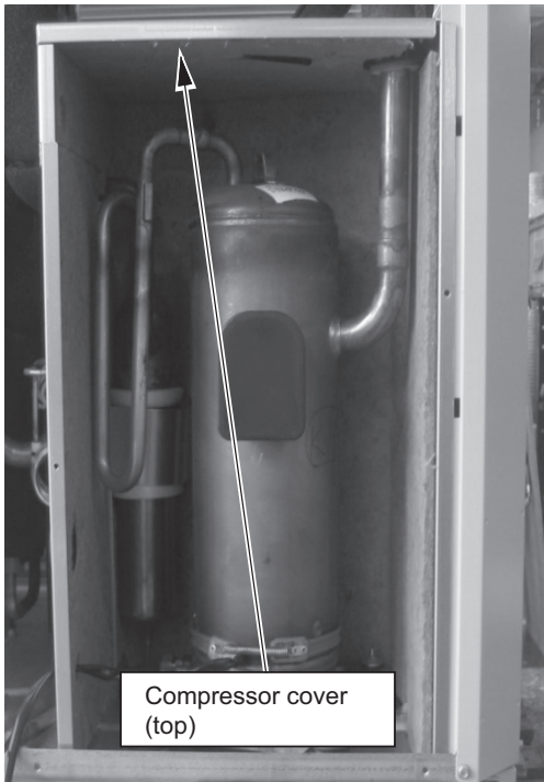
4. Remove the compressor cover (top).
