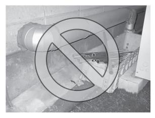
Store the pipes to be used indoors. (Warehouse at site or owner's warehouse) If they are left outdoors, dust, dirt, or moisture may infiltrate and contaminate the pipe.
