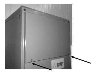
Step. 2 Remove the (1) screw that secures the panel to the air handler.
