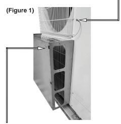
B. 2. Tighten the 2 screws already installed on the Front panel.
