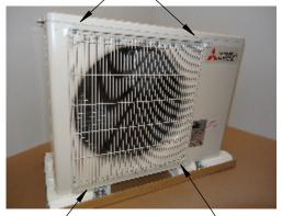
Remove the bottom screws and install the bottom bracket; reuse the screws taken out.
