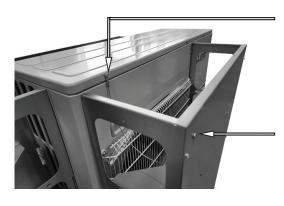
D. 1.Install provided Lanyards to cabinet chassis with the existing screws as shown with figure.
