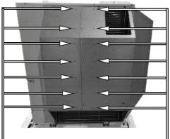
G. With the supplied #8 HWH SCREWS attach the RE RHS Panel to the RE LHS Panel using the provided holes. For best alignment and fitment work from Bottom to the Top when fastening the screws.
