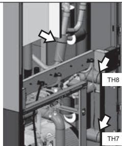
③ Remove the screw that is fixed to the I/O box (total 2 places), and remove the I/O box.
