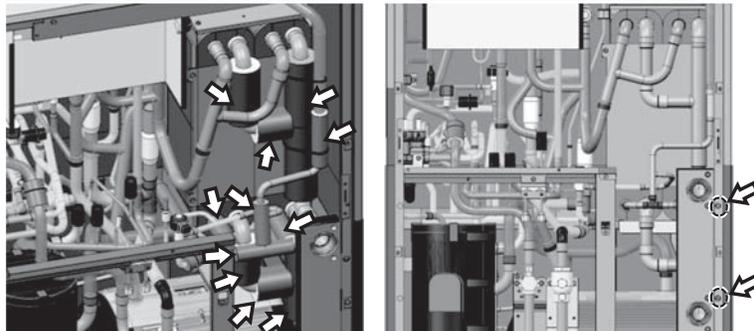
4) To remove the pipe from the Water Heat Exchanger
