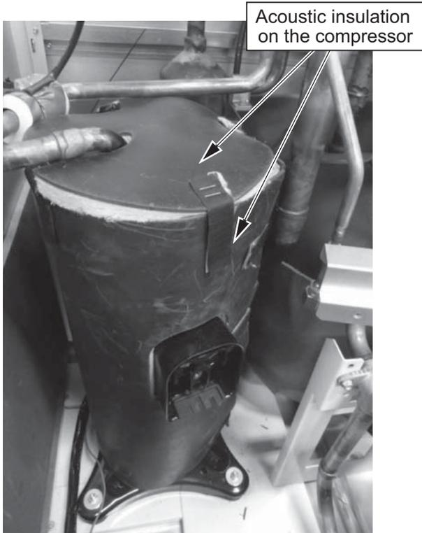
4. Remove the acoustic insulation from the compressor.
