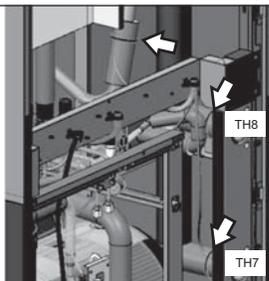
③ Remove the screw that is fixed to the I/O box (total 2 places), and remove the I/O box.
