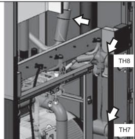
⑤ Remove the wire from cable strap on the Frame M.
