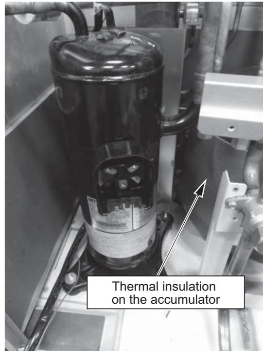
5. Remove or protect the wiring around the compressor and the thermal insulation on the accumulator, unbraid the pipe from the compressor, and replace the compressor.
