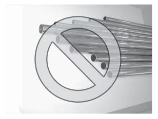
Both ends of the pipes should be sealed until just before brazing. Keep elbow pipes and T-joints in plastic bags.
