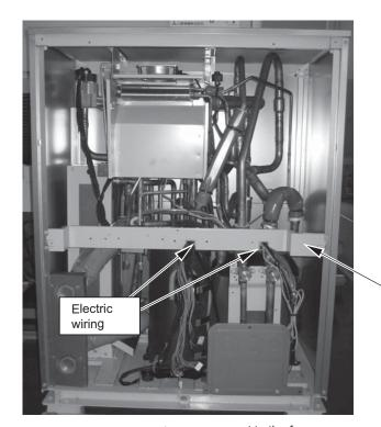
3. Remove the wires that are secured to the frame, and remove the frame.
