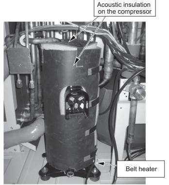
4. Remove the insulation material and the belt heater from the compressor.
