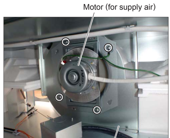
Motor fix plate
